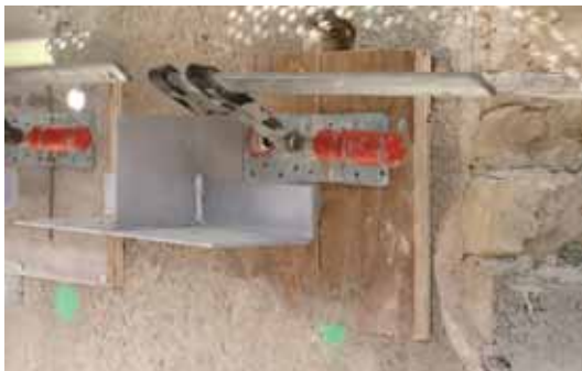
JMK+ P bracket assembly
