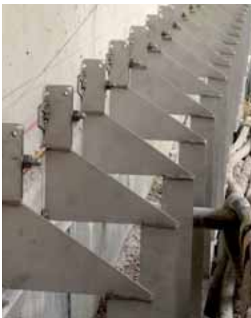
JVA+ NA as single brackets in normal wall areas
