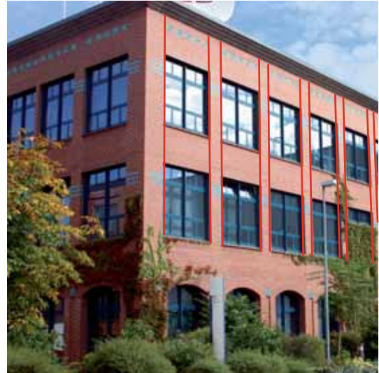
Continuous vertical expansion joints next to openings
